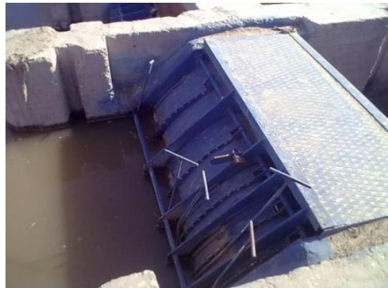
Fig. 3 A sample distributor of Neyrpic orifice module in Varamin Network
