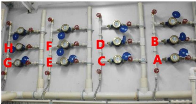
Fig. 3. Water Consuming Nodes and Leaking Points
