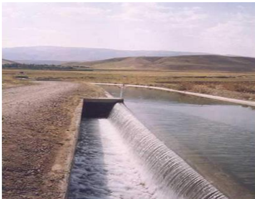
Figure 1. An example of side weir made on a channel with free flow surface [1]
