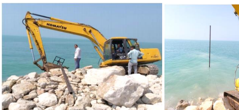
Figure 2. Index of settlement plates and erection at sea
