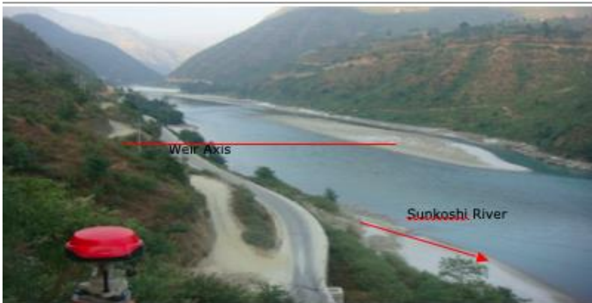
Figure 2. Weir axis at head works site
