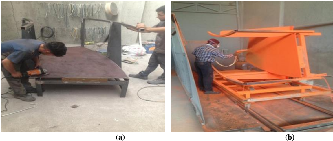
Figure 5. Stages of painting the channel modules: (a) sanding and removing the rust from the parts and (b) painting
